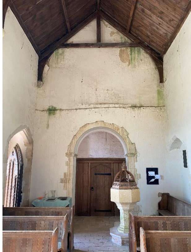
Figure 5 Inside looking West with the Font and Damp Walls
